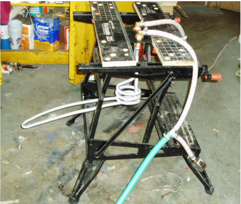
PRESSURE TESTING WITH HOT WATER
